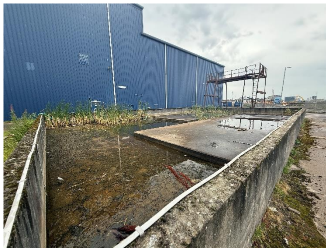
Image 16: Water tank which could be turned into a wildlife pond.
